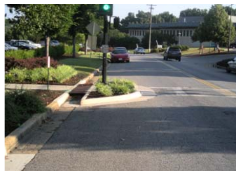
Example of curb extensions used around the Hospital in Lynchburg
